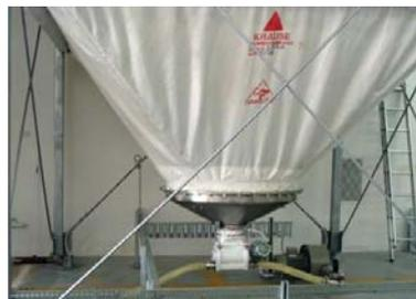
▲ 30t Krause Flexible flour silo fitted with vibratory silo discharger, Krause rotary feeder and connected to a Krause positive pneumatic conveying system.
